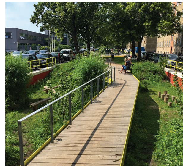
Raised walkway and stormwater storage system in Scandiagade, Copenhagen, 2021.
