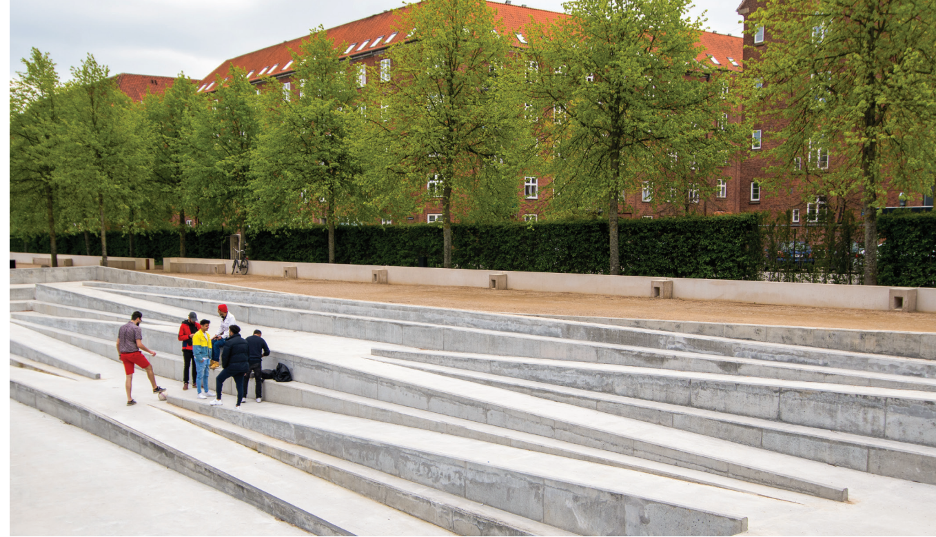
Sports arena and water storage system in Copenhagen's Enghaveparken, 2021.
